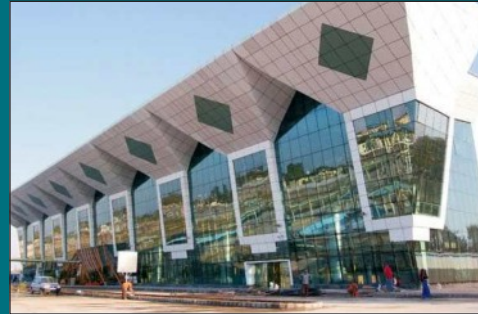
Maharana Pratap International Airport, Udaipur
